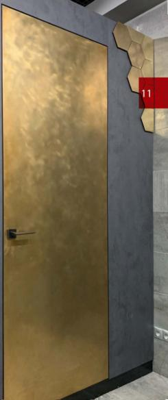
Frameless door leaf decorated with graphite mirror installed on concealed aluminium door frame and hinges. Construction made without TOP rail of the door frame.
